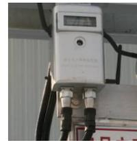
Figure 5. The picture of wireless MOA insulation monitoring node
