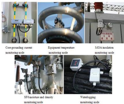
Figure 14. The scene photo of wireless monitoring nodes
